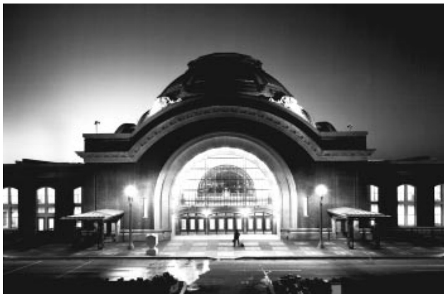
Tacoma's restored Union Station, which now houses courtrooms and offices of the U.S. District Court for the Western District of Washington, received an Honor Award from the National Trust for Historic Preservation in Boston in October.
